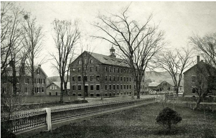
Faulkner & Colony mill soon after the Civil War
