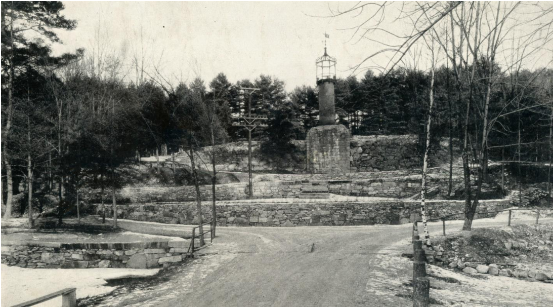
Robin Hood Park amphitheater, built by CCC work crews
